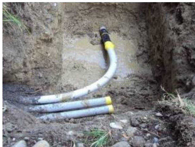
For the pulling in of the pipe a backreamer armed with carbide metal teeth \varnothing 115 mm (4.5") was used. Thanks to the power transmission by the direct-ram-principle, newly developed by TERRA AG, the pipe was pulled in easily through the hard soil.
