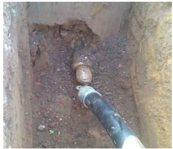
For the pulling in of the pipe a backreamer armed with carbide metal teeth \varnothing 115 mm (4.5") was used. Thanks to the power transmission by the direct-ram-principle, newly developed by TERRA AG, the pipe was pulled in easily through the hard soil.
