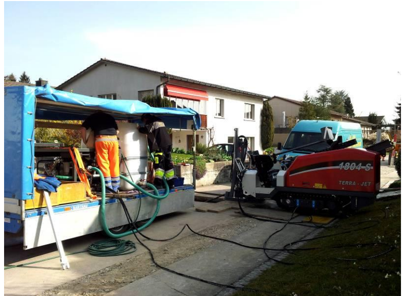
The mixing and pumping station, the drilling fluid tank and the tools are installed on the trailer. This allows easy mixing of the Bentonite into the drilling fluid.
