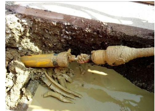
The backreamer arrives with a pipe in the starting pit.
